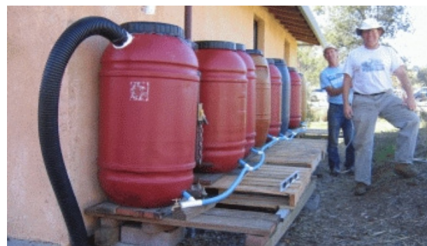
Daisy-chained system Courtesy of Acterra
