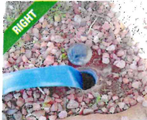
Sewer Cleanout Photo: Energy Master Pool Services
