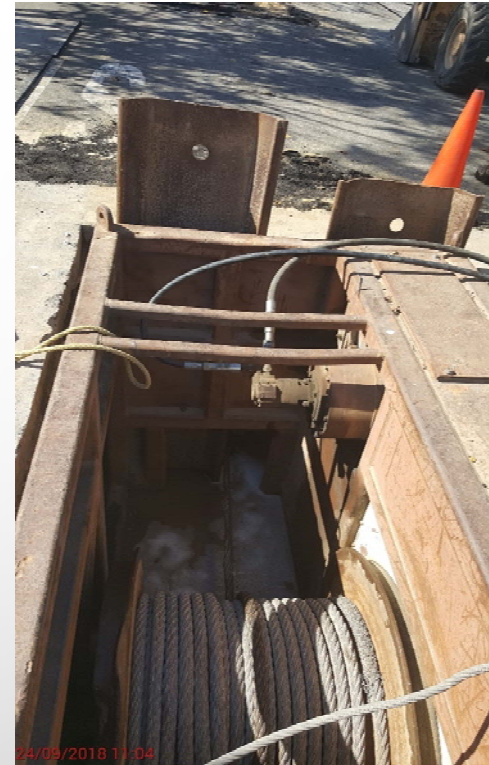
Figure 2. Winch Pulling Pipe for Bursting Operations
