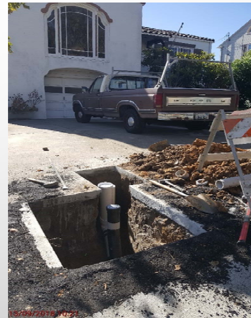
Figure 6. Sewer Lateral Cleanout and Backflow Preventer Installation
