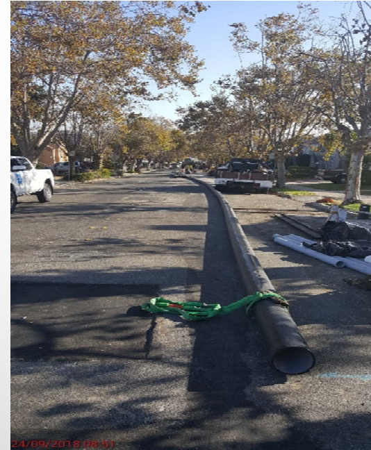
Figure 5. HDPE Pipe Prepared for Mainline Bursting
