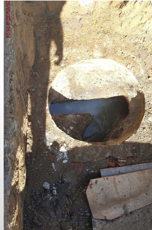
Figure 4. Existing Manhole Demolition for Replacement
