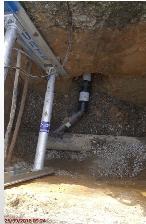
Figure 3. HDPE Lower Lateral Fused to New Main
