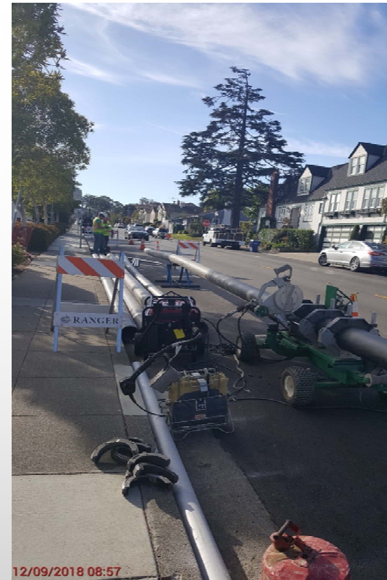
Figure 1. HDPE Pipe Fusing Operations
