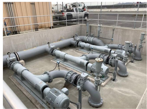
Figure 3 – Effluent Pumps
