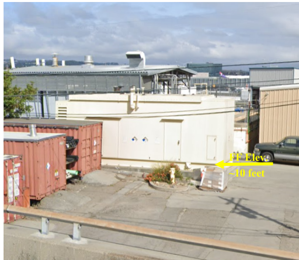
Figure 5 – Standby Generator Enclosure
