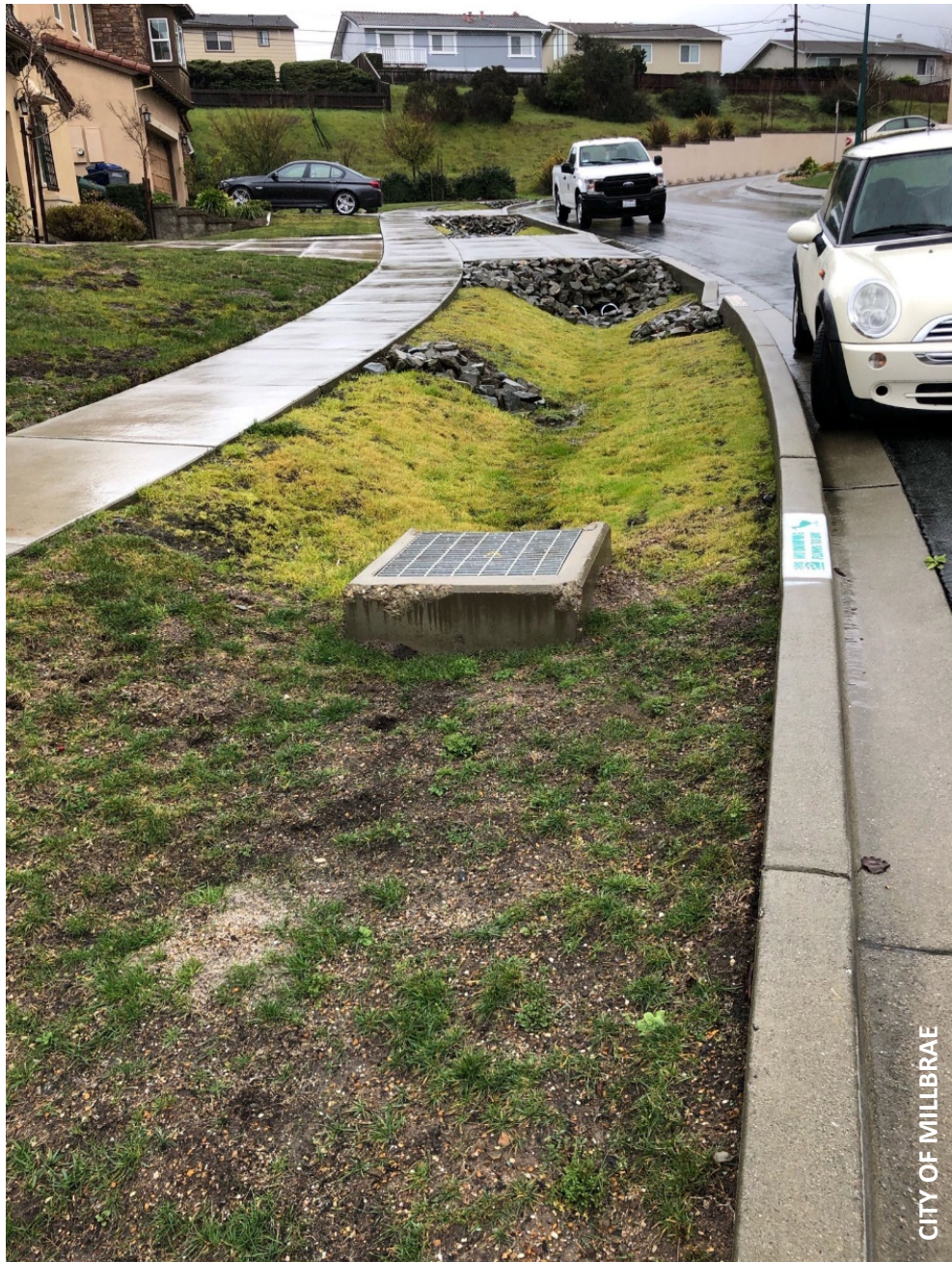
Bioretention area located at Millbrae Estates.
