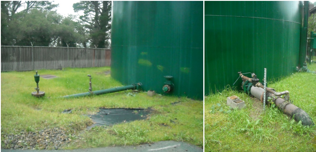
Figure 2.4.6 Helen Tank Piping Connections
