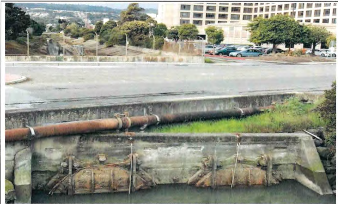
Photo 1-6. El Portal Canal Culvert Flap Gates at the Old Bayshore Highway
