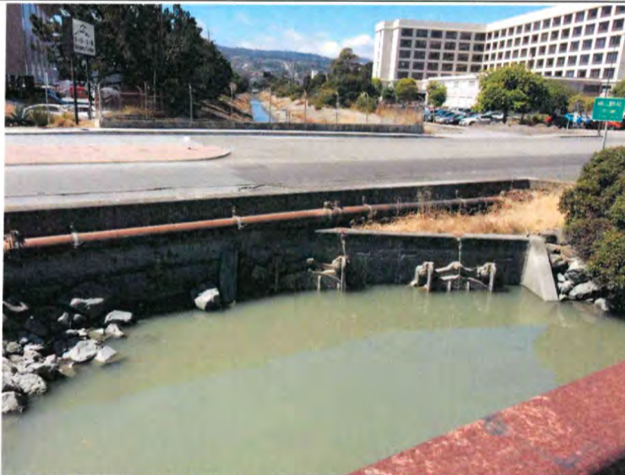
Photo 3-5. El Portal Canal Tide Gates, August 2017
