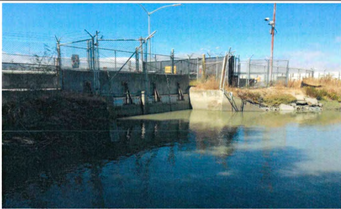
Photo 1-2. Highline Canal Box Culvert Flap Gates
