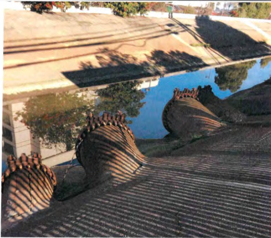
Photo 3-4. Cowan Pump Station Outfalls to El Portal Canal, December 2016
