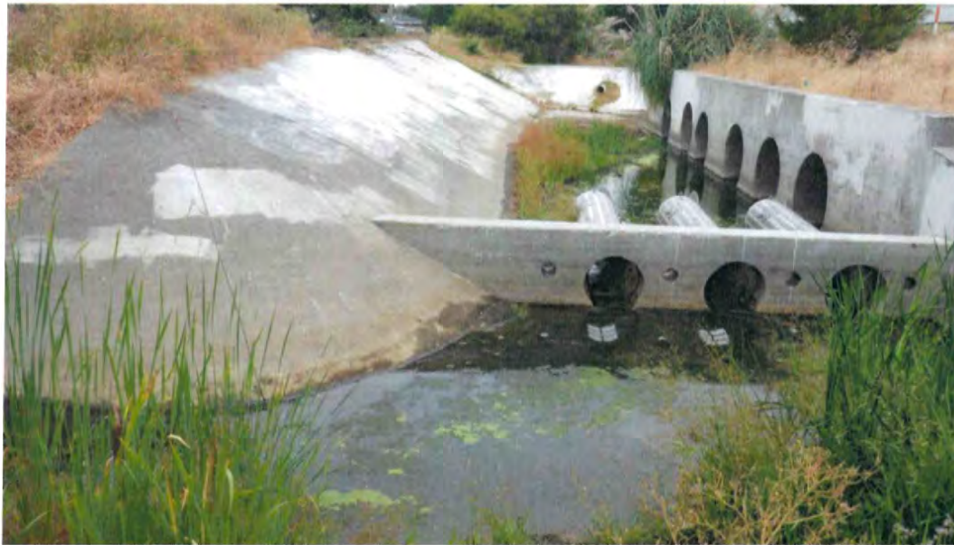
Photo 3-8. Landing Lane Bowl and Trash Capture Devices at Lomita Canal behind Landing Lane, August 2017
