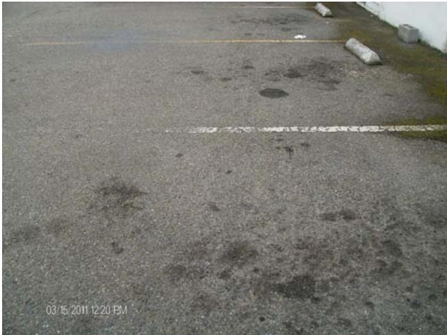
Photo 9: View of a typical oil stains observed in the asphalt parking area.
