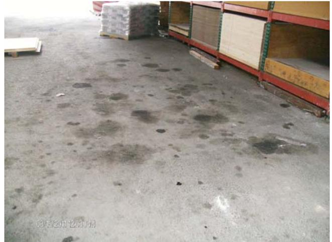
Photo 10: View of typical oil stains observed within the warehouse portion of 200 El Camino Real.
