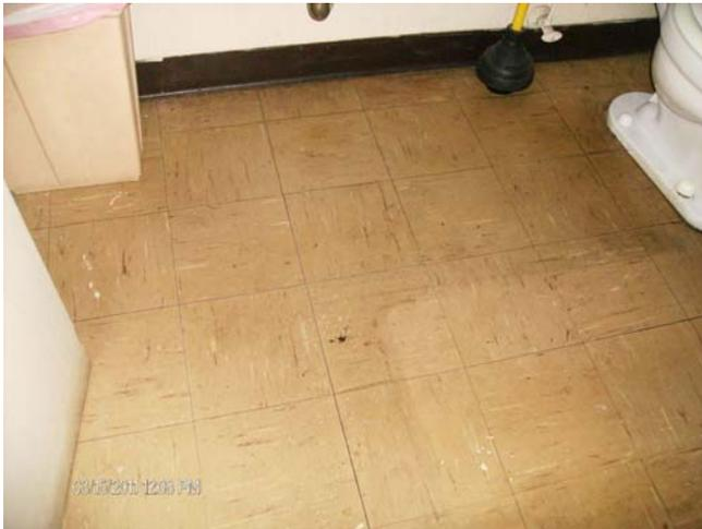
Photo 13: View of typical suspect asbestos-containing material observed in 200 El Camino Real.
