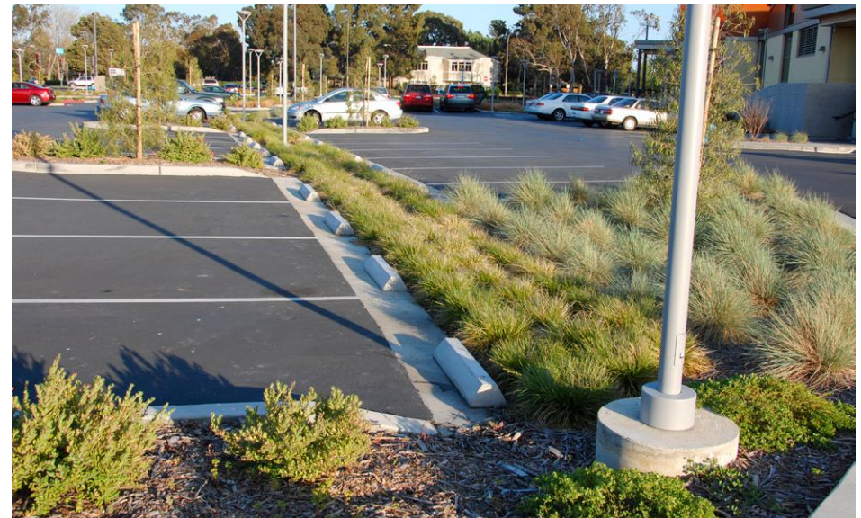
Stormwater management system in parking lots
