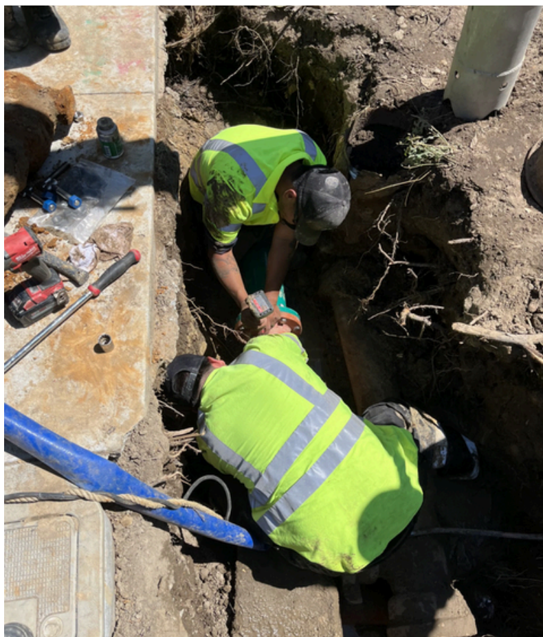
Michael Penagos and Saul Gonzalez working to repair a fire hydrant hit and damaged 07/27/25. The team installed new pipe, valve, and riser components to restore full service to the area.
